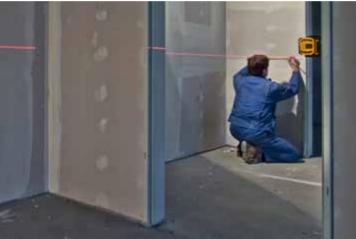
▲ Position the laser right where you need it. On the floor, stand, counter or connect to steel objects with the rare earth magnet on the back of the outer housing.
